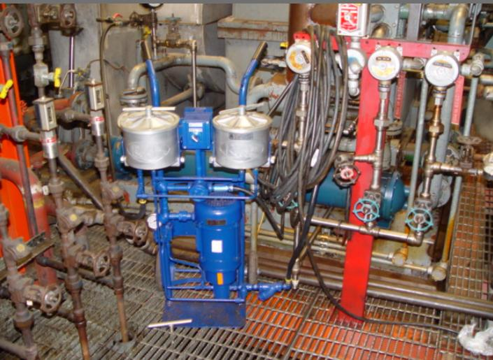
Off-line filter carts can be utilized for a variety of maintenance tasks in addition to the removal of oil contamination from systems while in operation.
